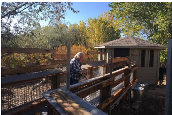
New plank fencing under construction - Steve Crouse
